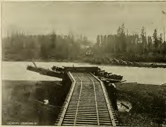
COMPLIMENT OF THE SEASONS CORLIAN RIVER BRIDGE, E. & N. RAILWAY, BRITISH COLUMBIA, RISEK SPAN 275 FEET LONG.
